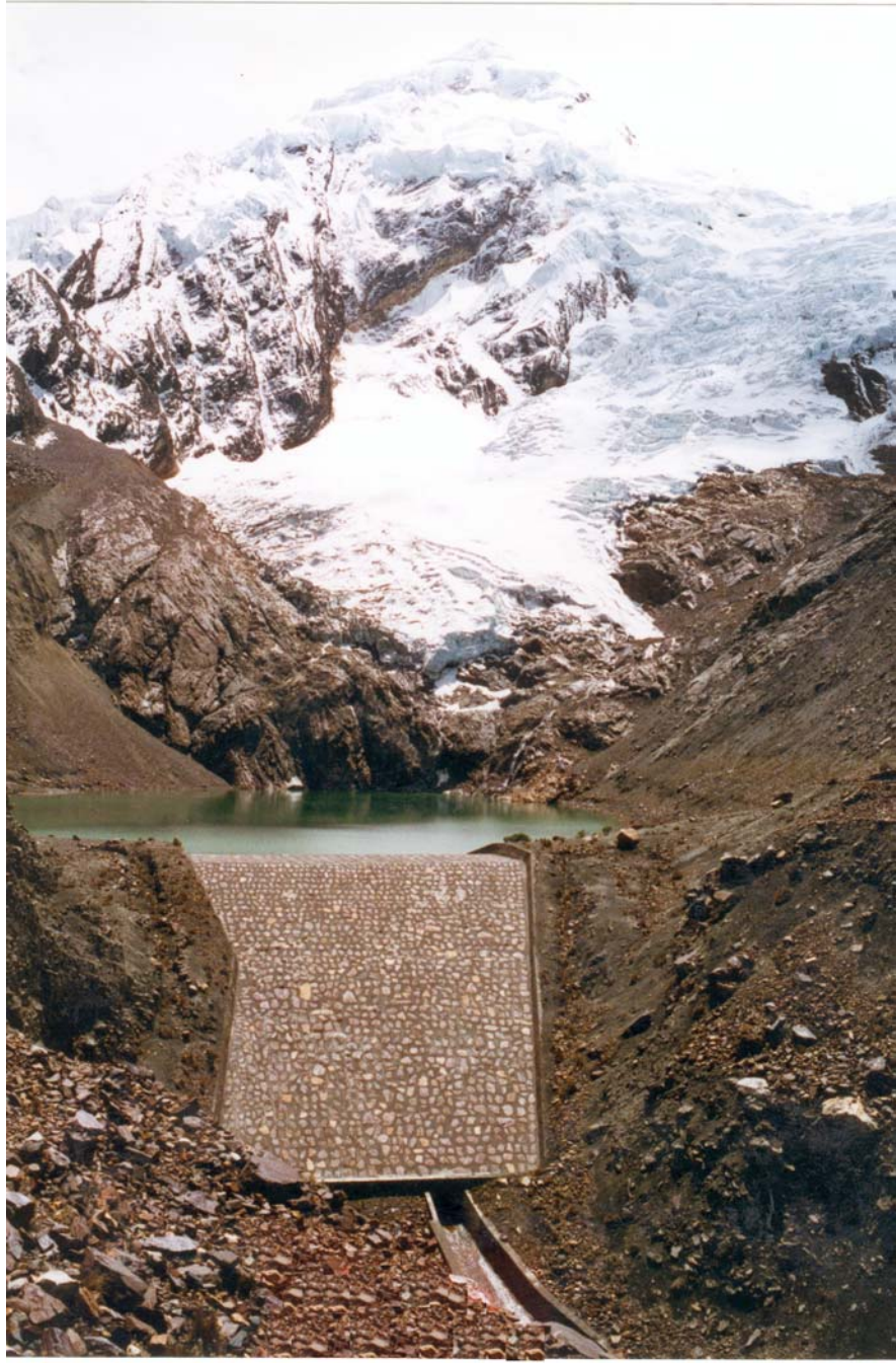
Figure 6. Example of a Lake Stabilization Project 64
